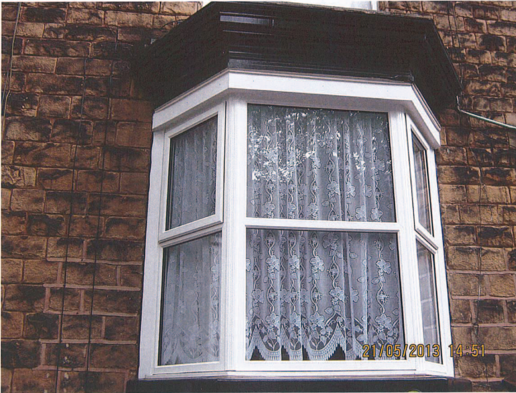
Appendix D - 23 Briar Road, close up of UPVC replacement window
